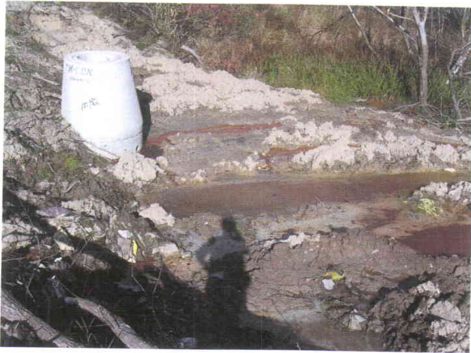
Photo 17 – Re-initiation of flow from Casselman Landfill at station CSW-1 (October 2004).
