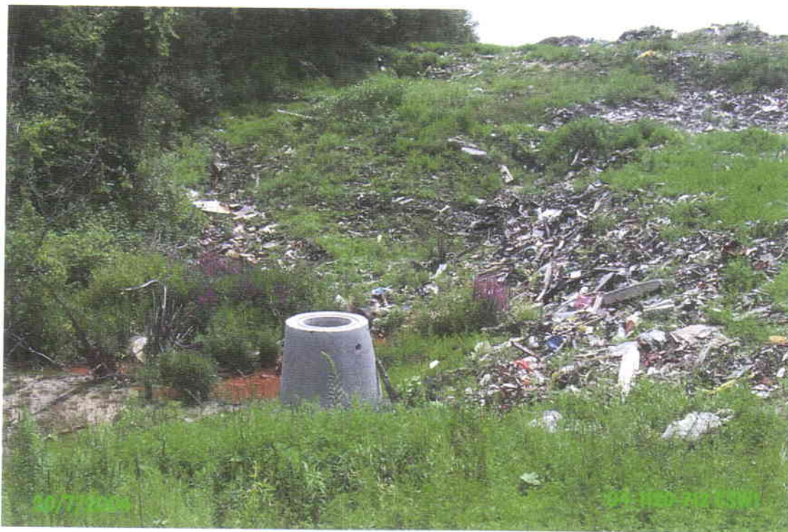
Photo 9 – Uncovered wastes at Casselman Landfill, before reshaping works (July 2004).
