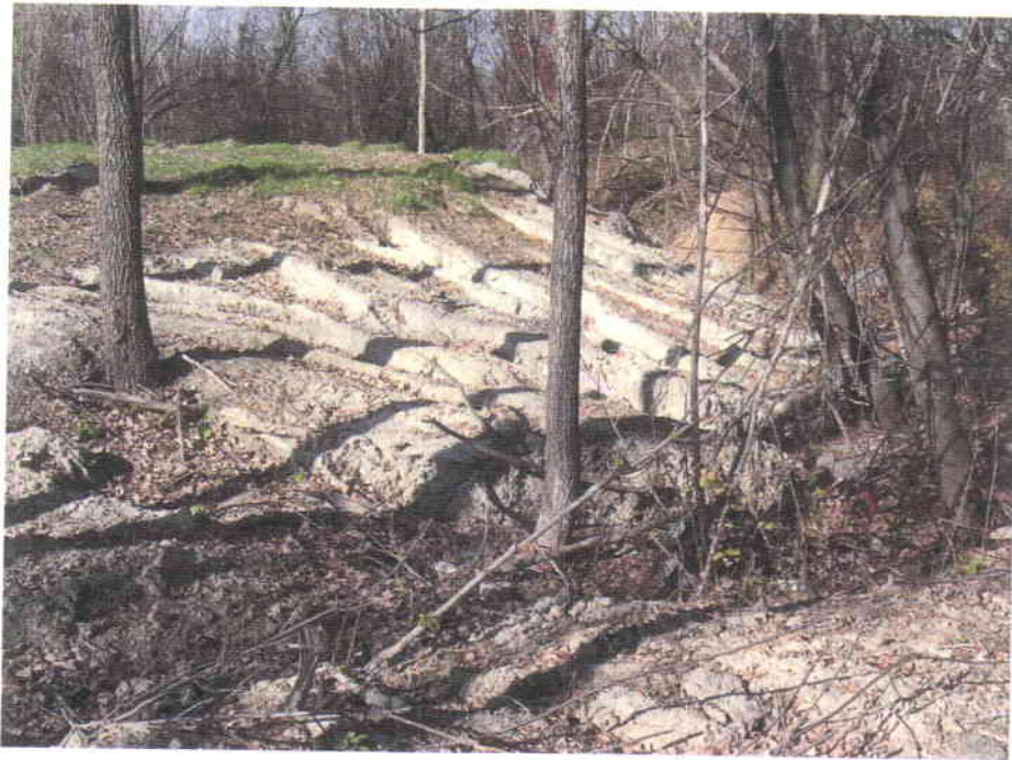
Photo 13 – Erosion channels, western edge of Ravine No. 3 (October 2004).
