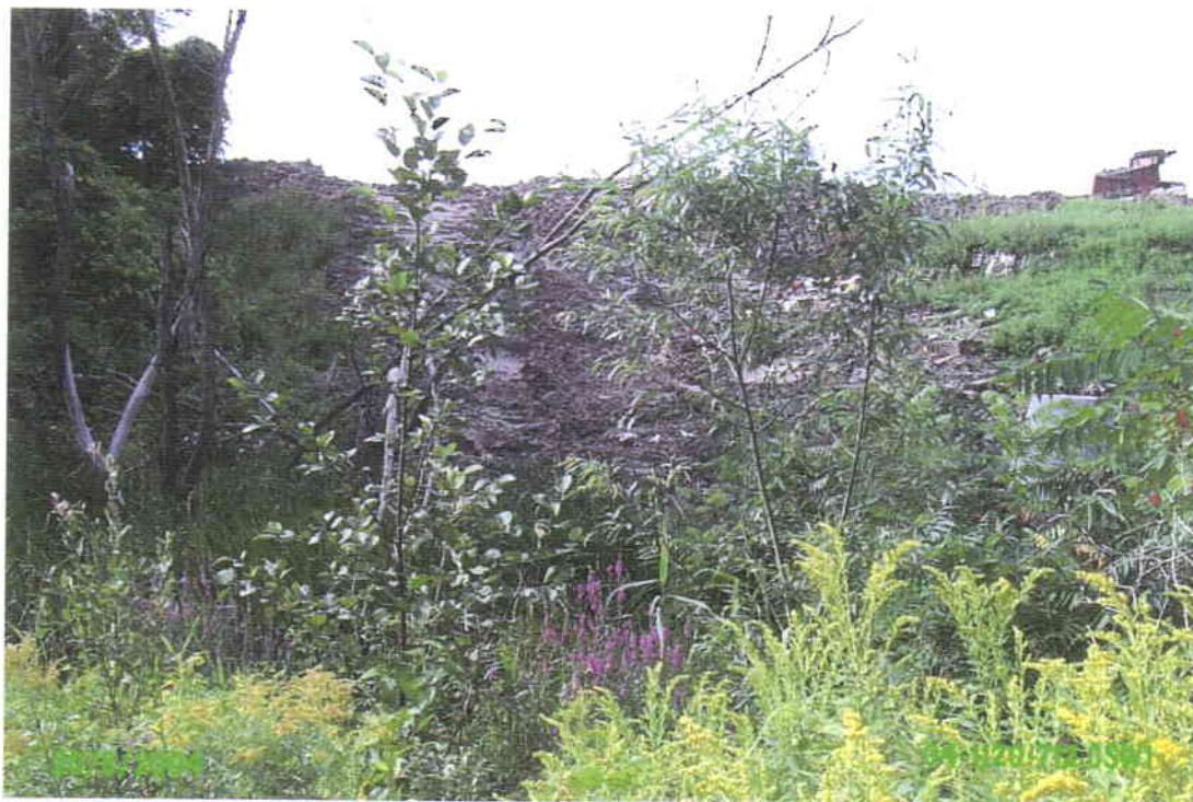
Photo 10 – Reshaping and covering works in progress, Casselman Landfill (August 2004).
